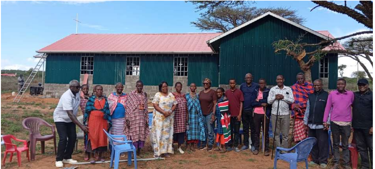
PCEA Ngujuka Church Construction
